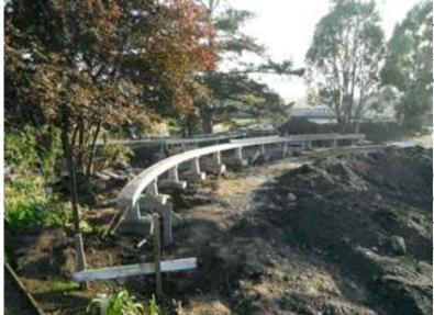
The curved beam section at the south eastern end will be poured on Saturday 21st, weather permitting and then boxing can be set up for the final curve section & bridge abutments along the eastern side. Mark is going to get a quote for rail steel for the extension - outside tracks will be 10 x 20mm and inside tracks 6 x 20mm flat bar.
